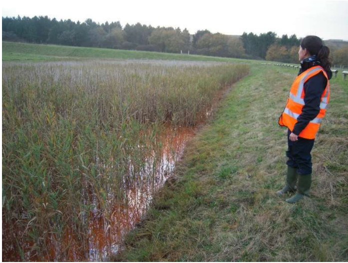
constructed aerobic wetland (coal mine drainage, north-east England)
