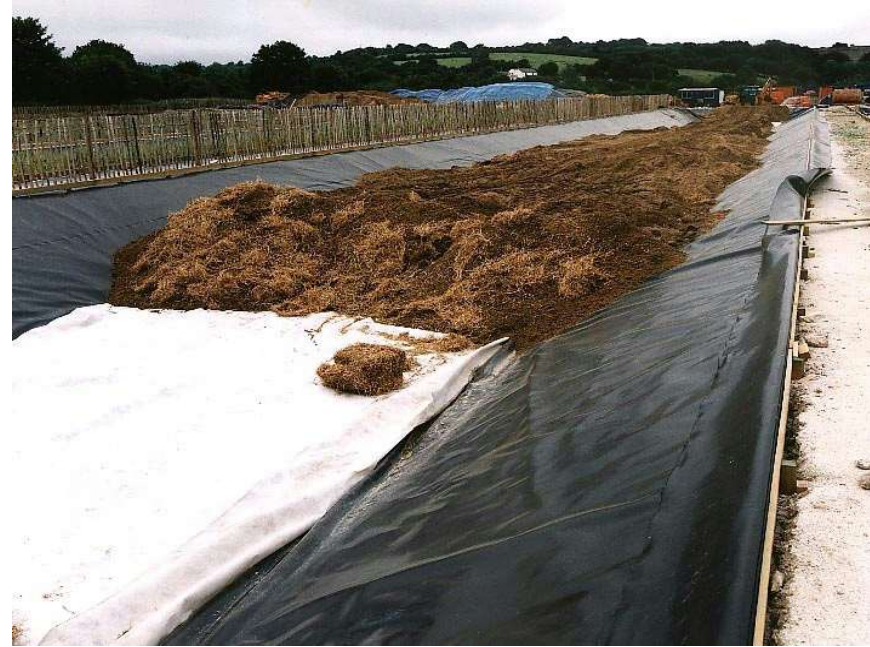
anaerobic compost "reactor" construction (metal mine drainage, south-west England)
