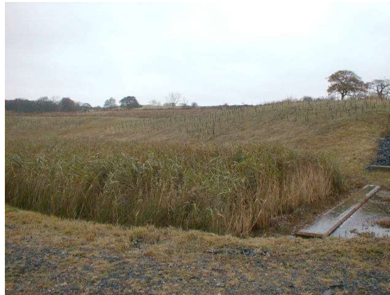
Chemical oxidation of ferrous iron in a surface lagoon
