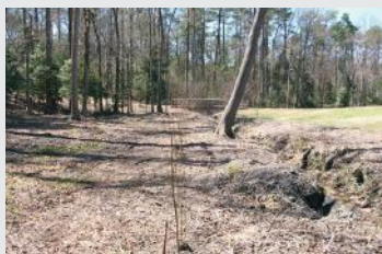
Phytoremediation Area B: Original installation – poplars and willows were installed to protect the surface-water swale visible on the right from contaminated groundwater.
