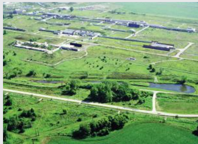
Line 1 Explosives Constructed Wetland: 2000 – created from excavated explosives impoundment
