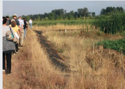
A subsurface gravel wetland cell treats wastewater vertically. A pipe in the center brings the effluent to the surface which is treated as it slowly flows down through gravel to the bottom of the cell.
