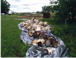
Barrels of pesticides (Dinoseb) excavated from the site. The pesticides had leached into the groundwater, polluting local drinking water supplies.
