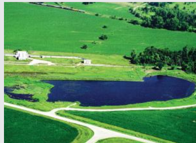
Line 800 Explosives Constructed Wetland: 2000 – created from excavated area of explosives
