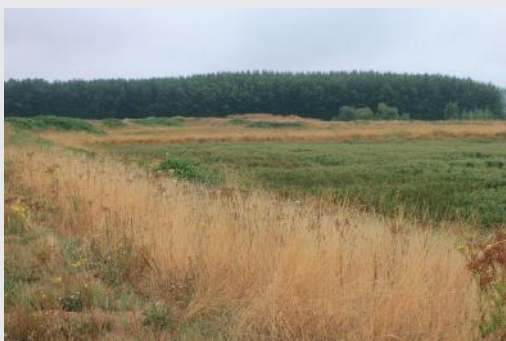
Effluent storage lagoon in foreground will be converted into an irrigation regulation reservoir for temporary storage and constructed wetland for effluent cooling. Poplar tree stand, visible in background, blends well with the surrounding rural agrarian landscape.
