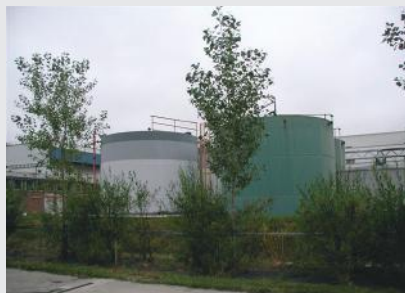
New poplar and willow buffers were planted around above-ground storage tanks in 2006 to create a preventative remediation buffer for any potential future releases.
